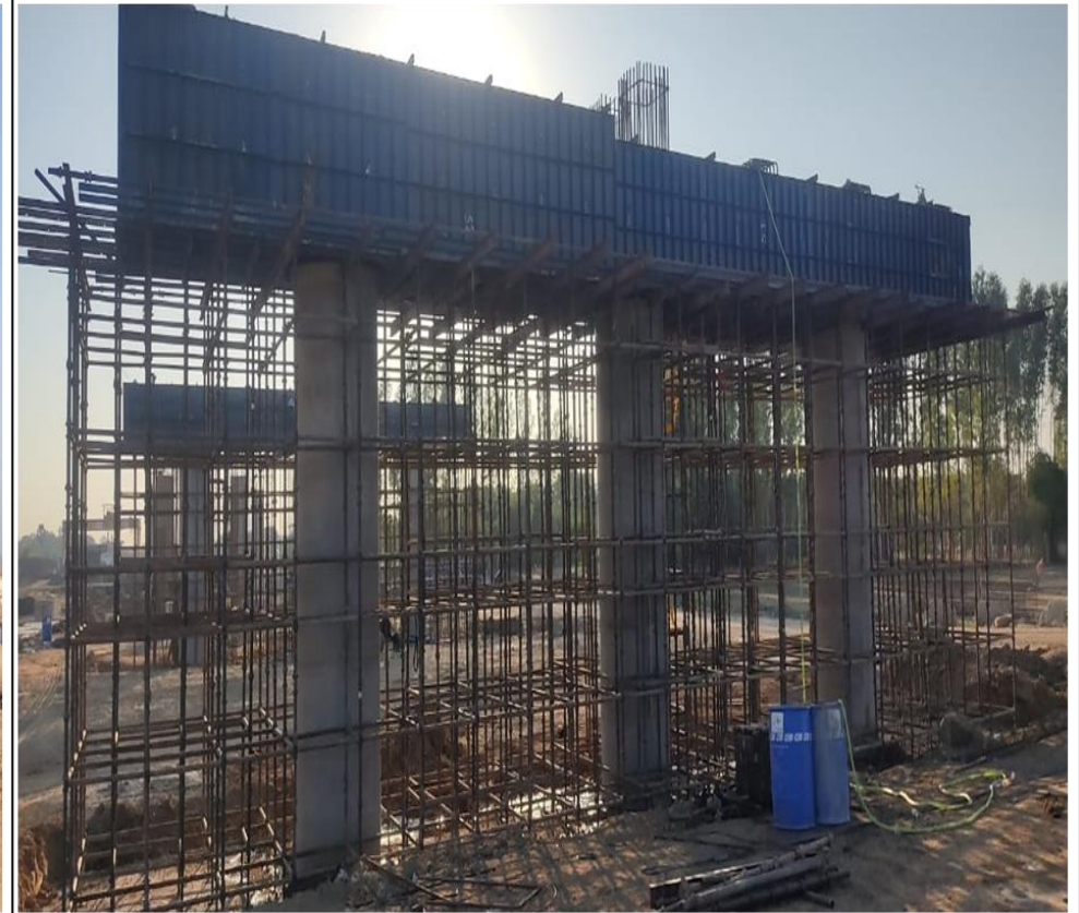
Curing on Pier Cap P-4, RHS A-1 side MJB @ 352+281
