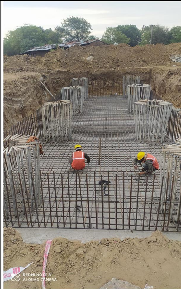
Pile Cap reinforcement binding at MJB 352+281
