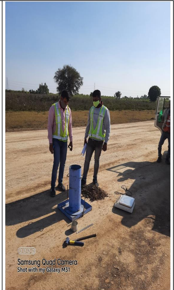
SG top fdd at ch.-360+ 600 to 360+ 720 LHS
