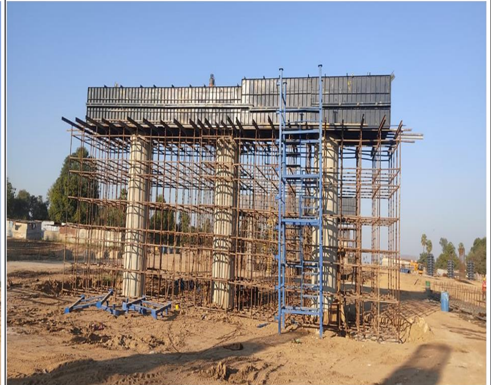
Pier Cap –P-5 RHS A-1 side MJB @ 352+281
