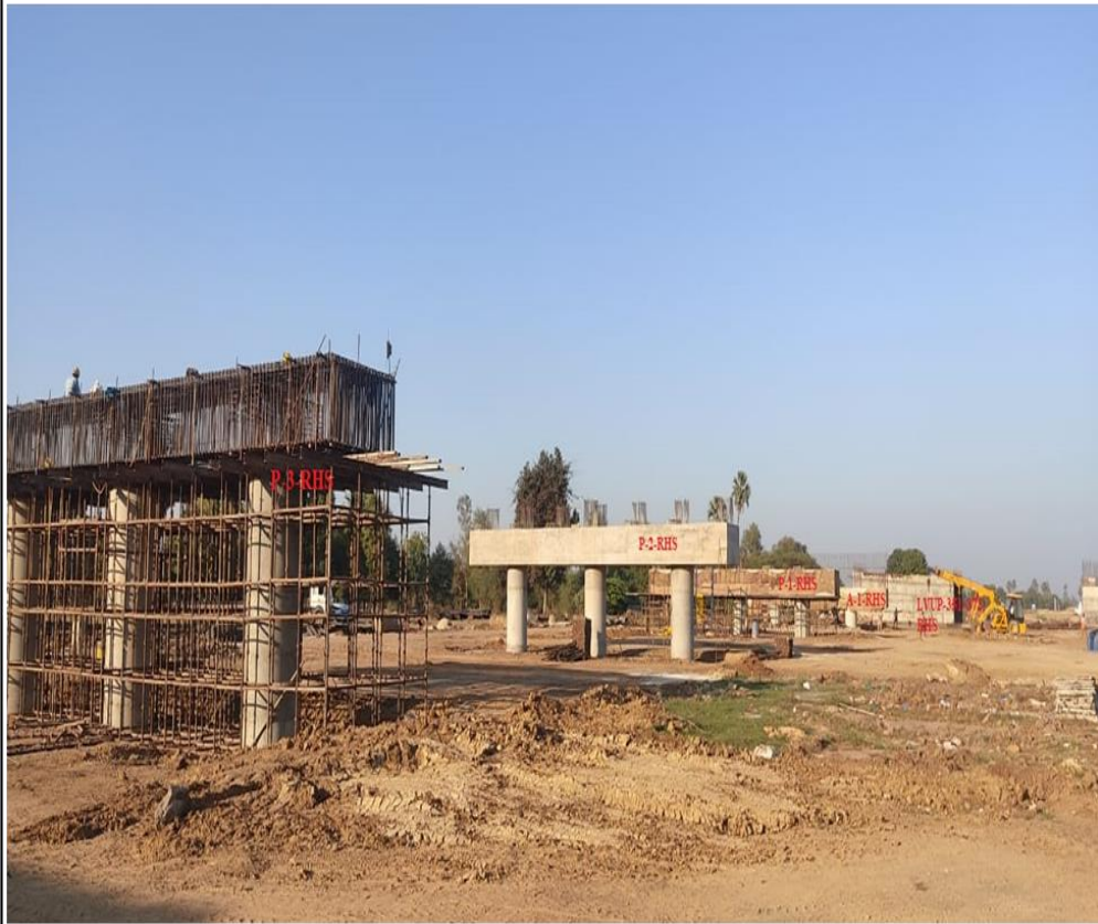
Pier Cap –P-3 reinforcement fixing & Pier Cap A1,P1,P2, RHS A-1 side MJB @ 352+281
