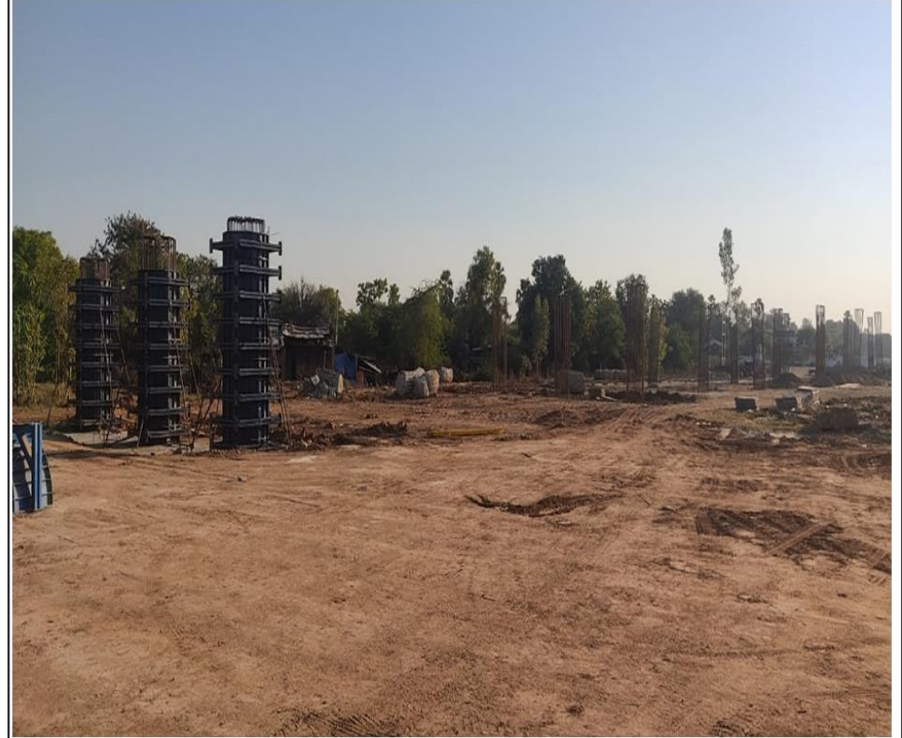
Pier Shaft A1 side LHS MJB @ 352+281
