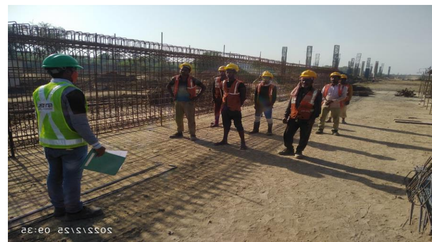
TBT conducted at A2 site at girder casting yard ch.352+281
