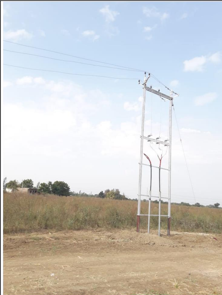
Utility Shifting- Electric line charging at ch.362+650
