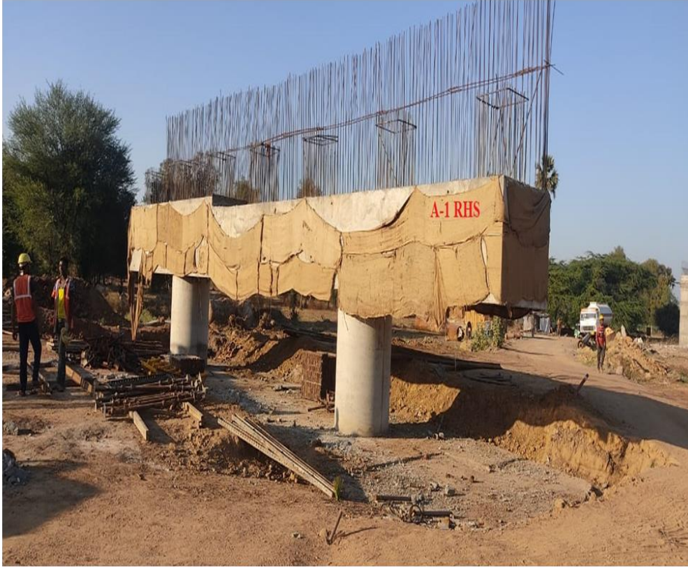
Abutment Cap –A-1 RHS A-1 side MJB @ 352+281
