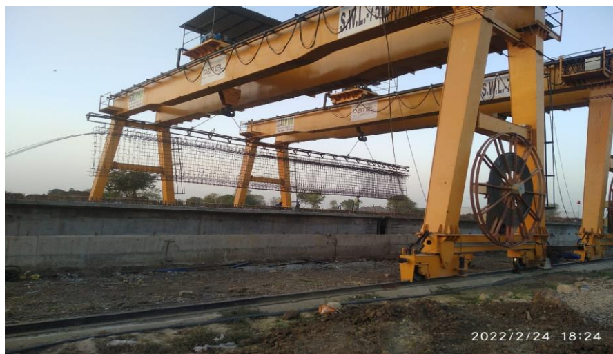
Girder cage shifting at girder casting yard
