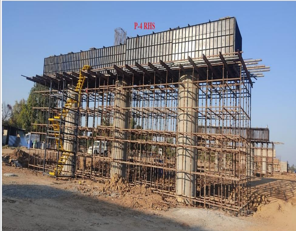
Pier Cap –P-4 RHS A-1 side MJB @ 352+281
