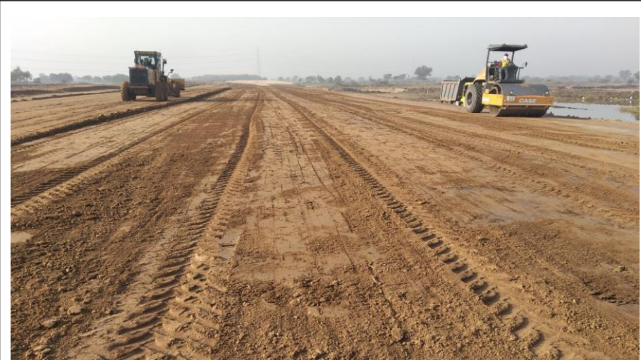
EMB TOP Grading and rolling RHS
